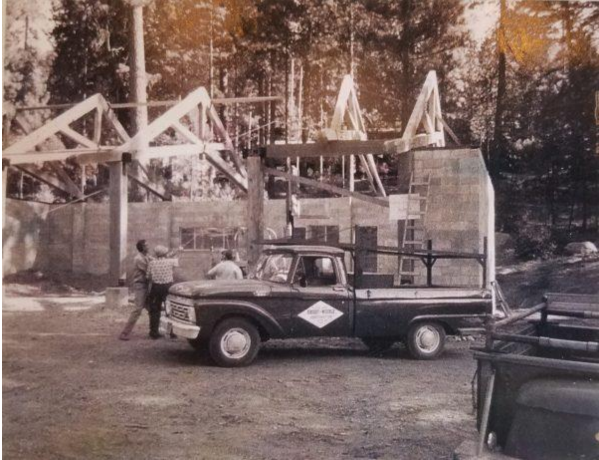
Building the firehouse. Photo courtesy Lilburn R. Prather.
